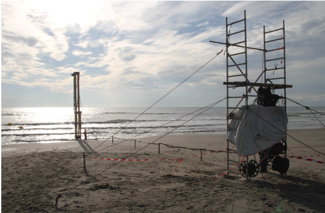
Figure 3.1: Photograph showing the experimental setup and their location on the upper part of Rousty beach. The TLS was fixed on the 4.8 meters-high tower standing on the left part of the picture while the scaffold is on the right. The buried sensors can be observed in between.
